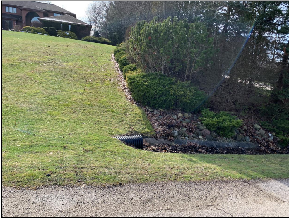
PHOTO NO. 31: Springer Drive, Facing South near Address 8130, Concrete Swale with Leaf Litter
