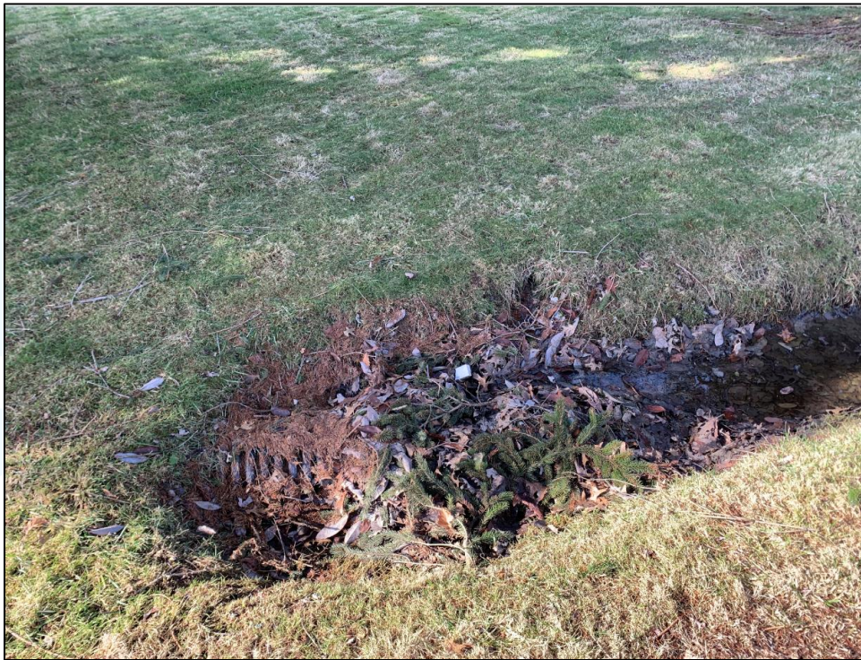
PHOTO NO. 8: Beechwood Drive – Drainage Swale with Plant Debris
