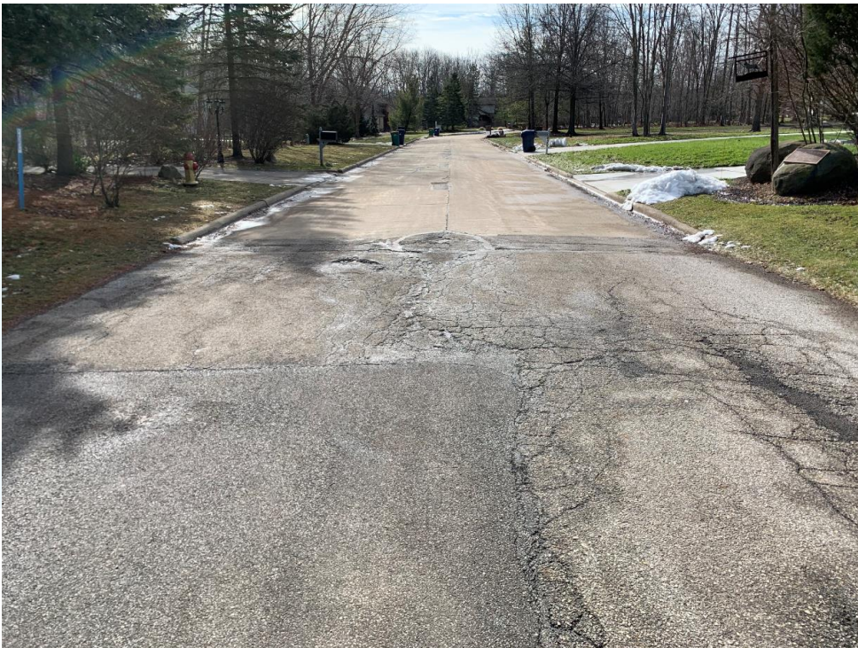
PHOTO NO. 18: Crestwood Drive, Facing South near Address 10870, Transition from Asphalt to Concrete Surface
