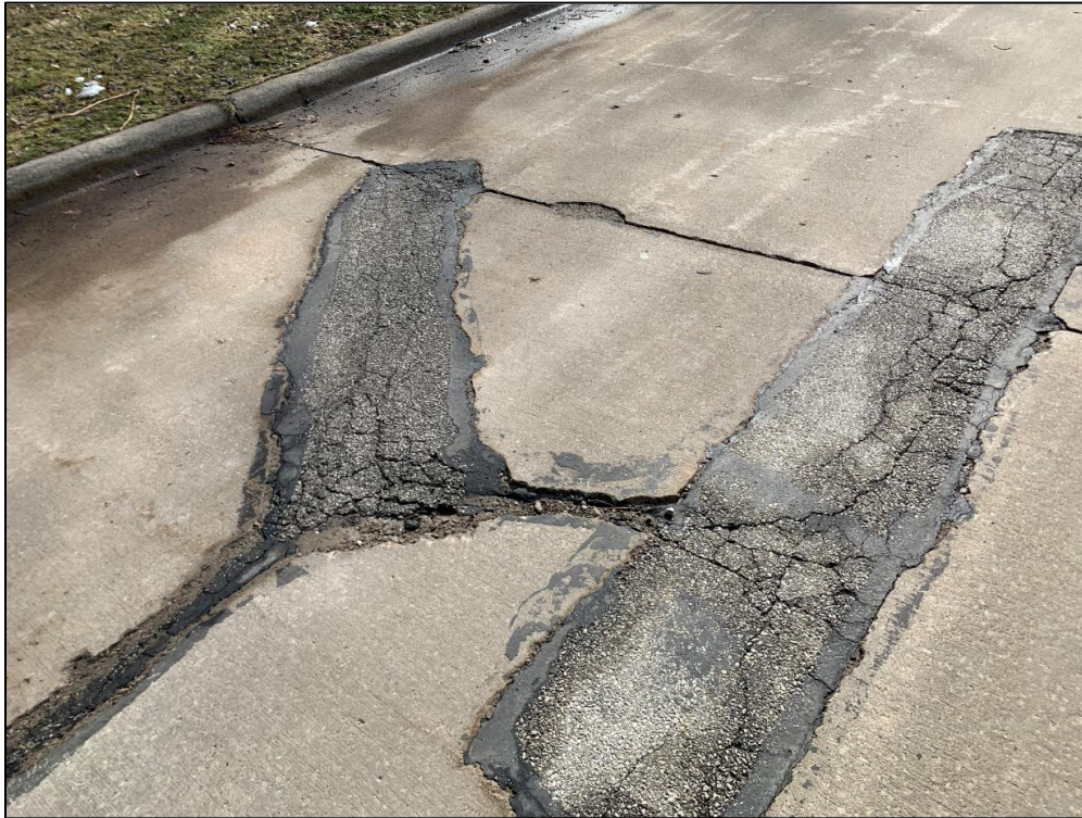
PHOTO NO. 19: Crestwood Drive, Crack and Joint Repair
